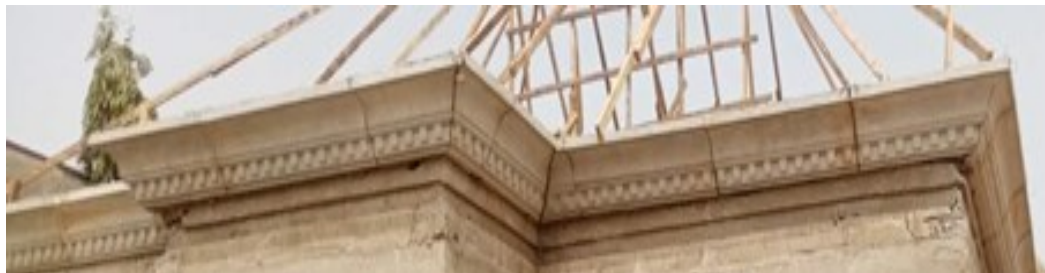
Figure 1: Parapet wall after construction
